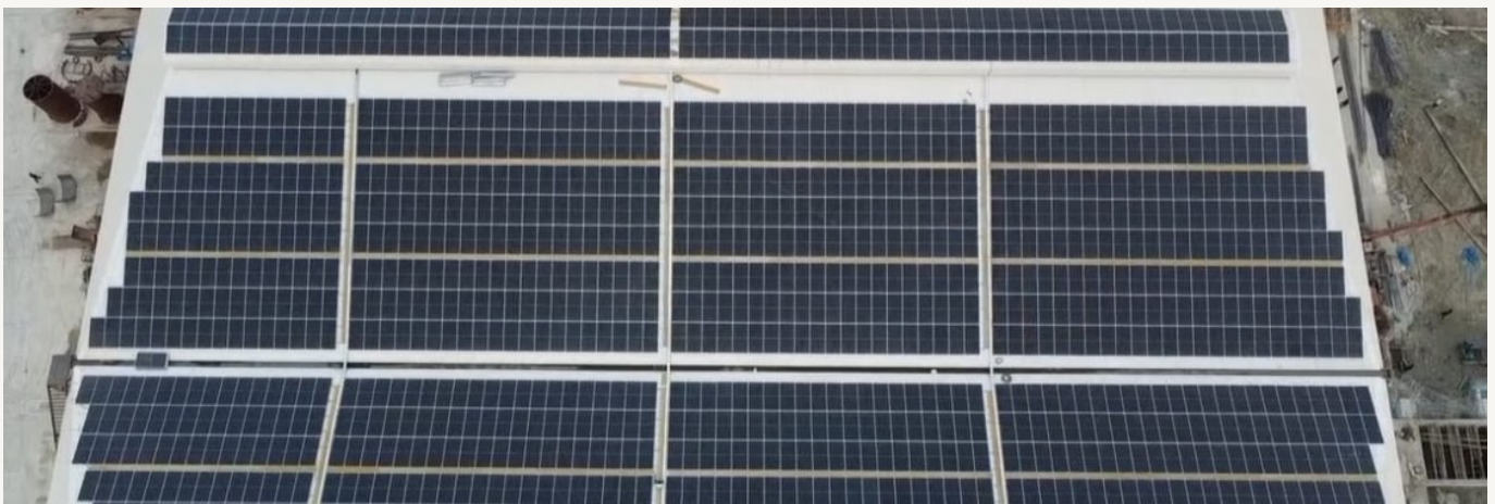
Akij Agro Feed rooftop project - Vvon portfolio
